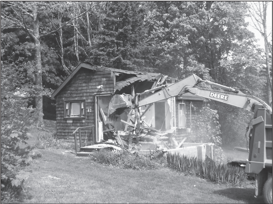
Tearing down the house. In a day it was all over.
