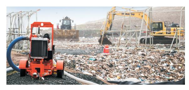
A recent Saturday at Cell 7B, Otter Lake Landfill's working face, shows idle machinery awaiting the start of the workweek. The white metal screens, vaguely resembling hockey nets, are portable litter fences that move in conjunction with bulldozer operations to protect against flying debris. On windy days, the litter fences are vital.
